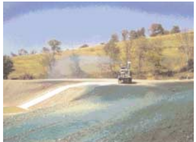
A manure storage pit, an important agricultural best management practice, being hydroseeded by Tioga SWCD.
